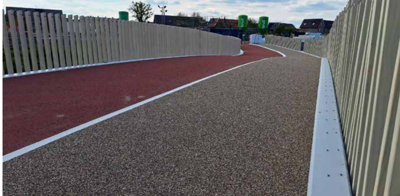
Composite Bridge in Barneveld
